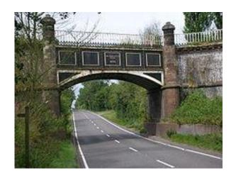
A short cast iron canal aqueduct between Stretton and Brewood and near to Belvide Reservoir. Designed by Thomas Telford and bearing his name and date of construction 1832. It carries the Shropshire Union Canal 30 feet above the A5 at a skewed angle,
